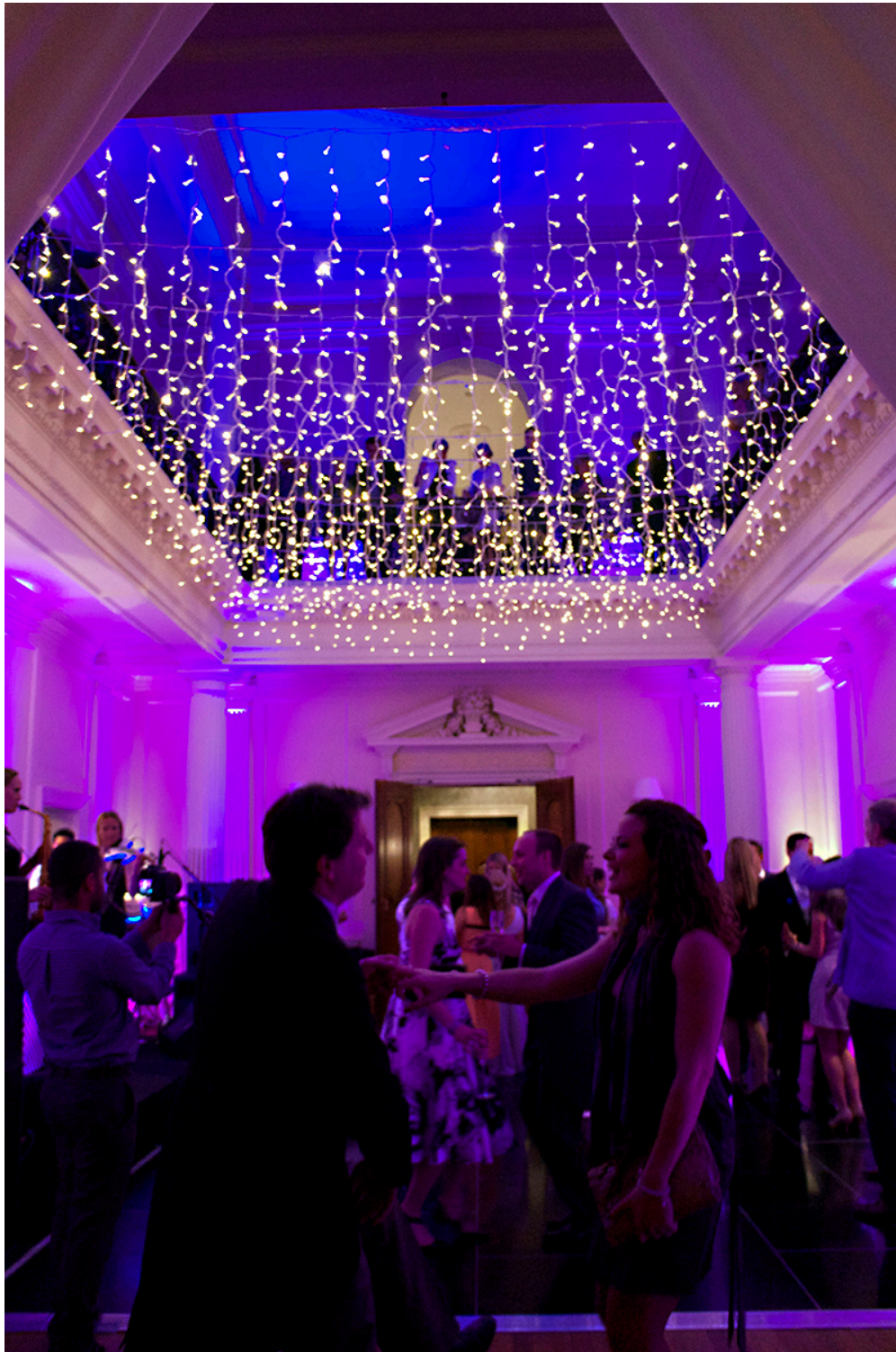
Pea Light Installation From Side to Side of Balcony
